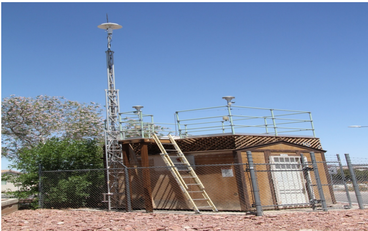
Figure 128. Green Valley monitoring site (street view).
