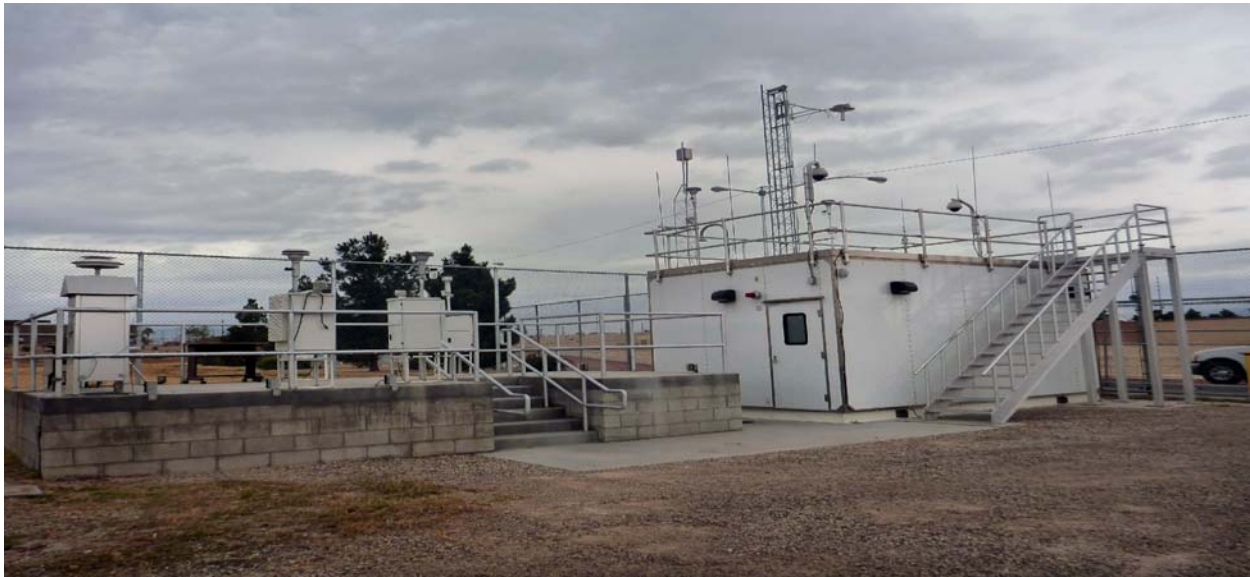
Figure 108. Jerome Mack monitoring site (street view).
