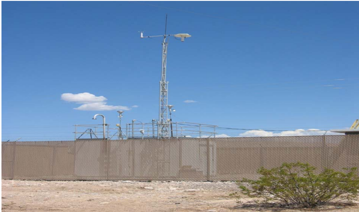
Figure 145. Jean Monitoring site (street view).
